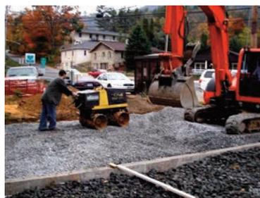
**Figure 23:** Compacting the open-graded aggregate base (Source: NCSU-BAE).
