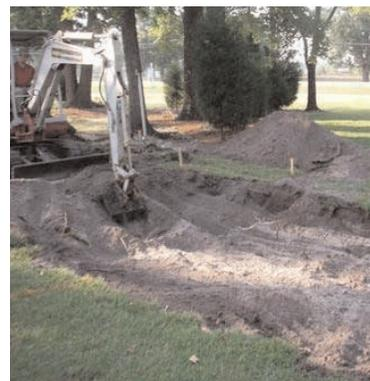
**Figure 17:** *Where possible, excavate soil from the sides of the pavement area to minimize subgrade compaction from equipment (Source: NCSU-BAE).*
