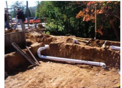
**Figure 21:** Installation of upturned underdrain and observation well (NC 2012, p:27).
