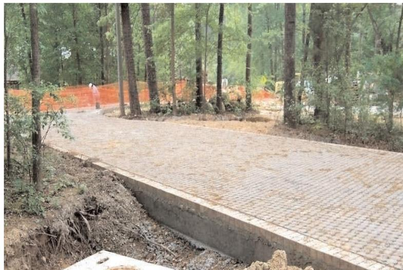
Figure 11: Edge restraint (Source: NCDENR).
