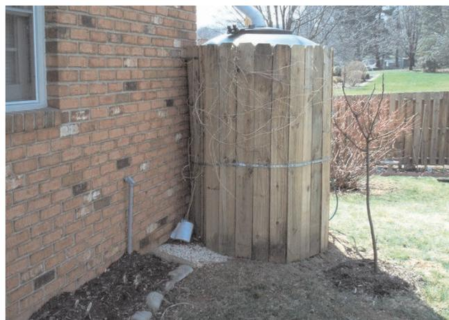
Figure 3: Residential Nonpotable System – Roanoke VA (Source: VADCR, 2011).
