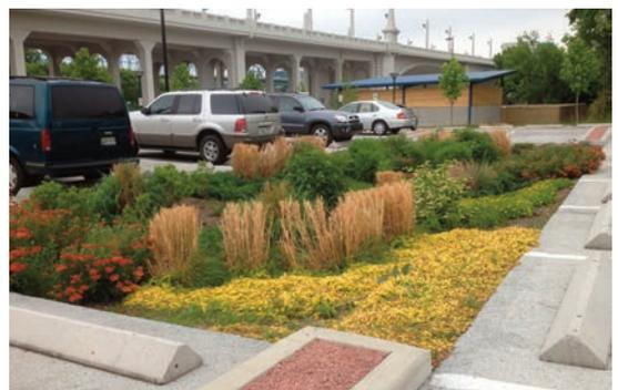
**Figures 2 & 3: roof leaders are directly connected to the bed. Bioretention that manages runoff from a parking lot (Source: The SMART Center).**
