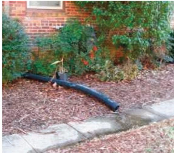
**Figure 4: Poorly designed and installed downspout disconnections (Source: Carmen, NCSU).**
