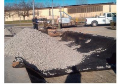
**Figure 20:** Filter fabric is installed on bottom and sides of reservoir layer (Source R.K.).
