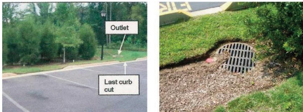
Figure 15: Short circuiting in bioretention (Source: VADCR).
