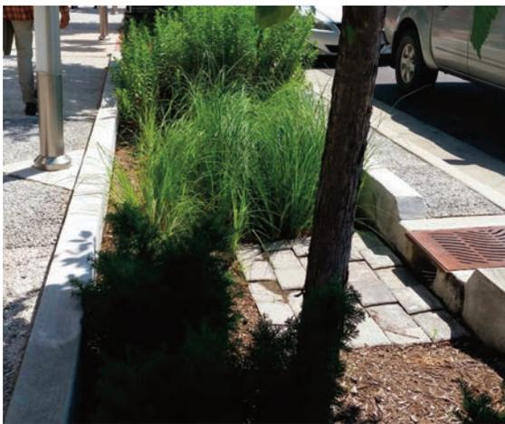
**Figure 2: Street side planter boxes. runoff enters the planter boxes through curb cuts
