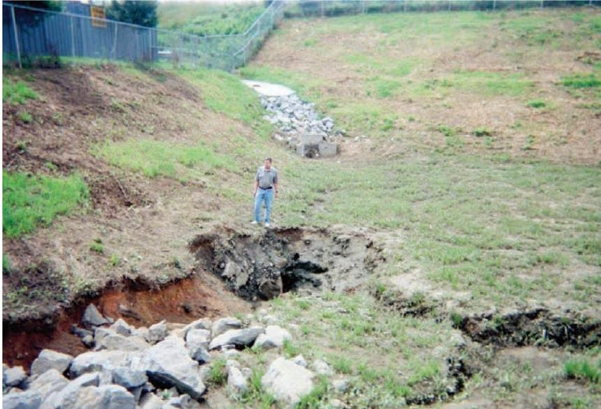
**Figure: 7.1 Sinkhole Collapse in SCM.**
