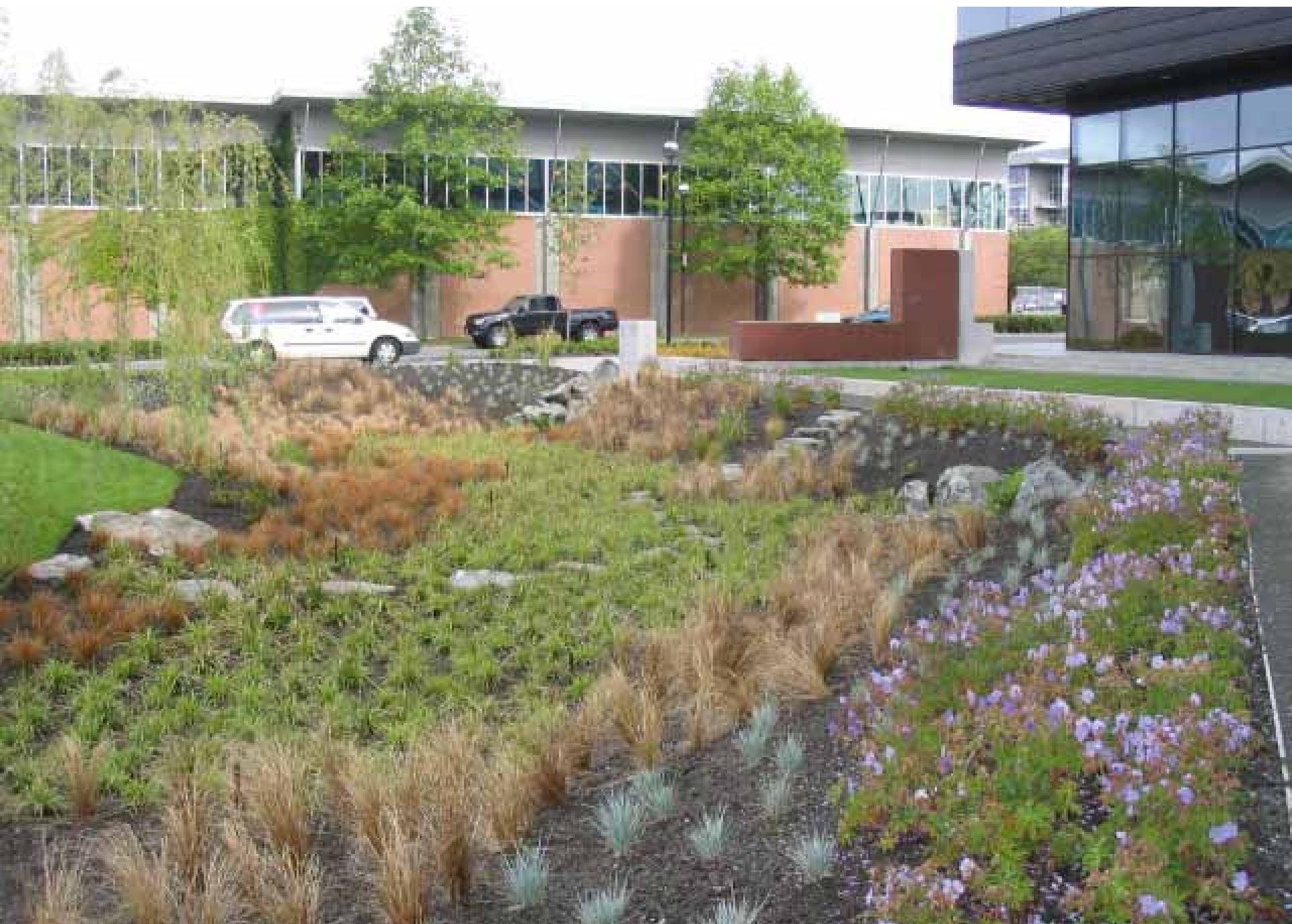
Storm Water Detention Garden/ Bioswale
