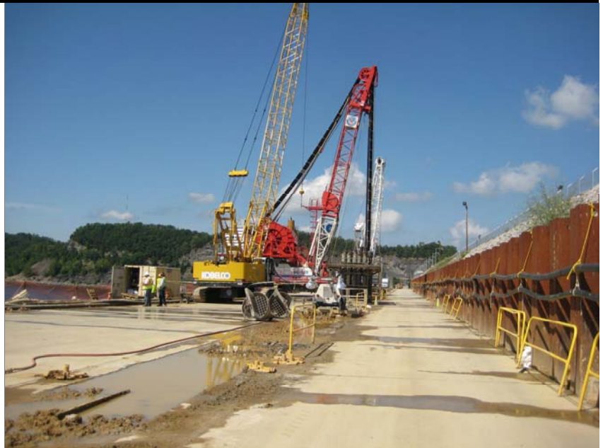
Above: Hyrdomill drills on the platform at the Wolf Creek Dam.
